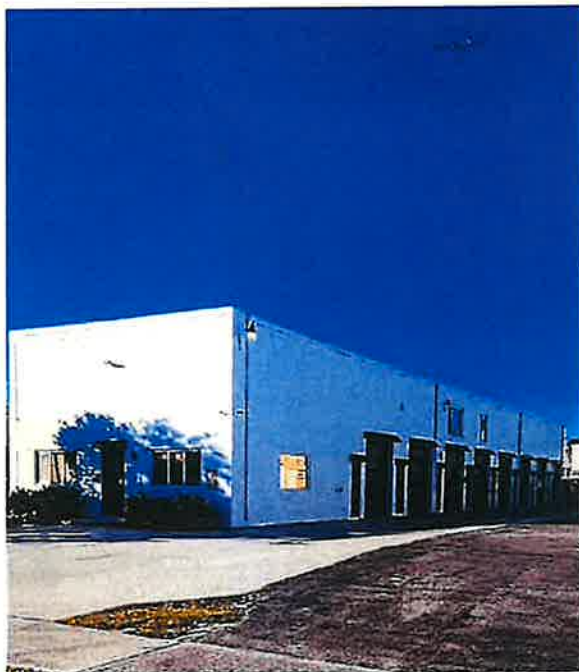
Figure 4 - 1343 S Killian Front Facade
